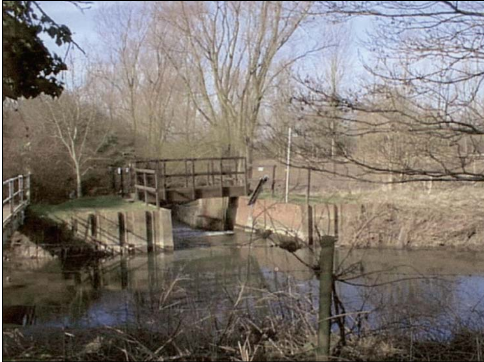
Site Prior to Installation
